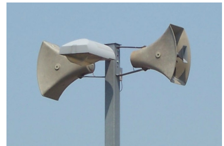
Figure 25.15: These speakers are shaped to take advantage of diffraction for sound waves. The narrower the opening, the wider the diffraction pattern. The speakers are designed to diffract sound waves horizontally, where they can be heard by people on a train platform. Photo credit: A. Duffy.
